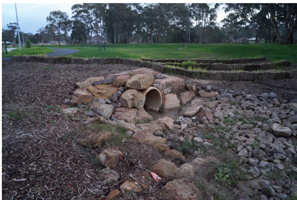
Figure 1- Well designed stormwater outlet
