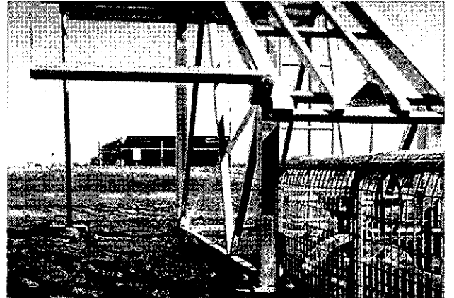
Wimmera Mallee Water Another view of Pumping Station
