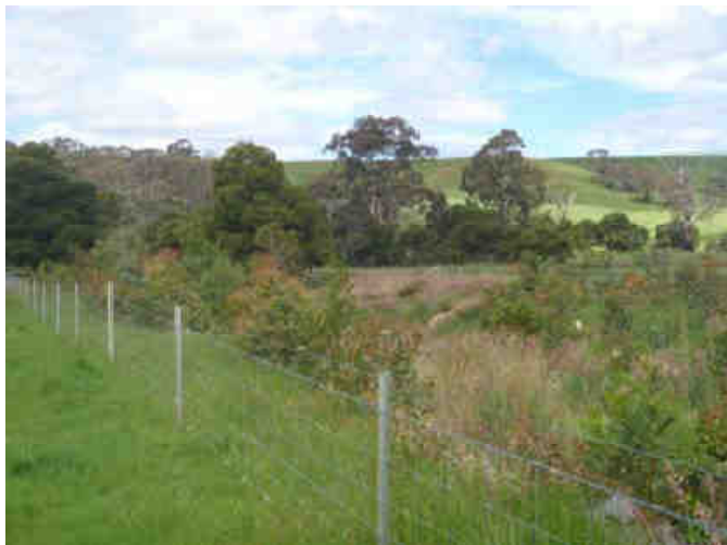
Site after waterway protection works were completed, Coliban River tributary near Trentham, November 2010.
