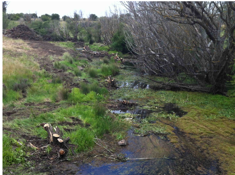
Willow removal works are progressing near Windmill Bridge.
