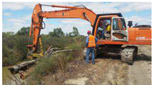
Installing the snags in Pyramid Creek
