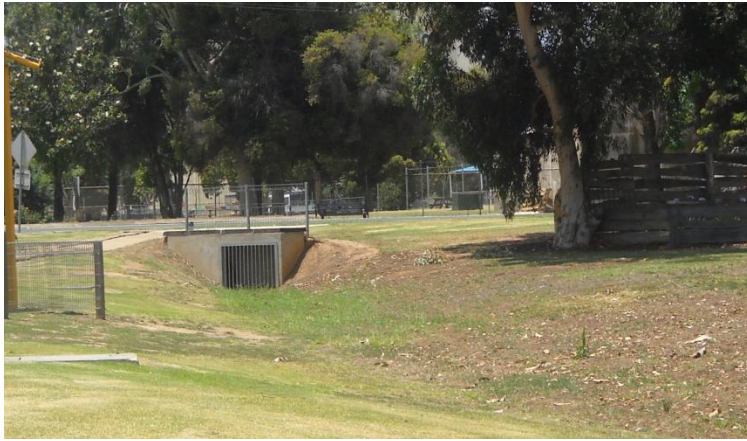
Park – Victoria St/Northern Hwy - Drainage pipe behind bar screen
