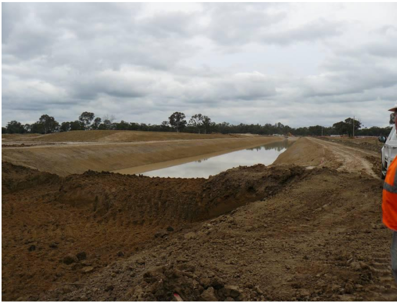
Photo 2: Hipwell Road Channel with rainfall runoff, June 2013.
