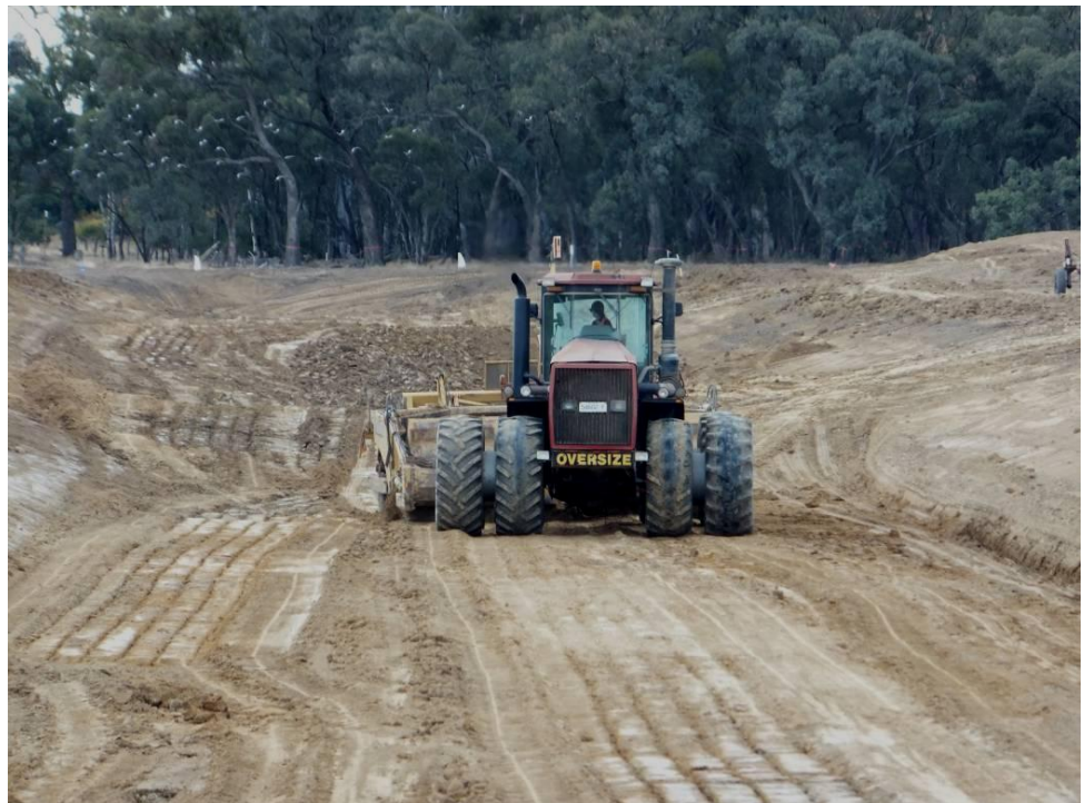
Photo 1: Scrapper working to excavate Hipwell Road Channel.
