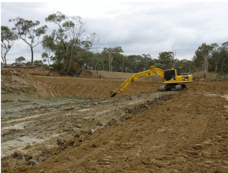
Photo 4: Cofferdam in Gunbower Creek
