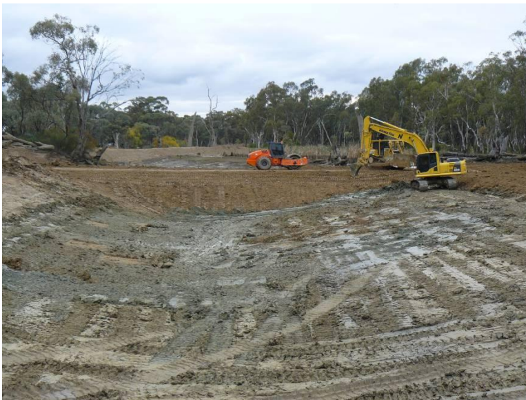
Photo 3: Cofferdam in Gunbower Creek
