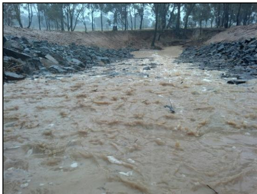
Figure 2: A repaired erosion control structure near Tarnagulla performing its role of reducing the in-stream gradient and preventing further streambed incision, June 2013.
