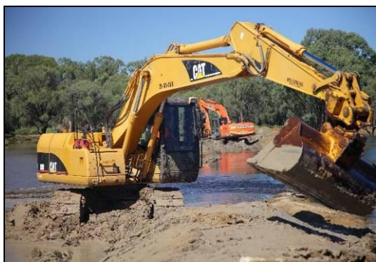
Figure 9: An emergency levee repair, January 2011
