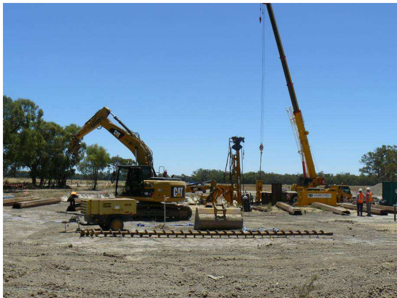
Photo 2: Construction activity at Hipwell Road.
