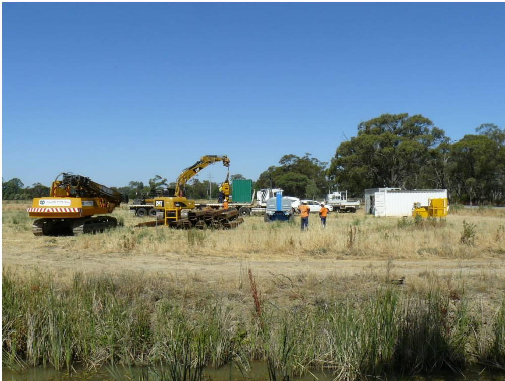
Photo3: Construction crews mobilising to site in December 2012.
