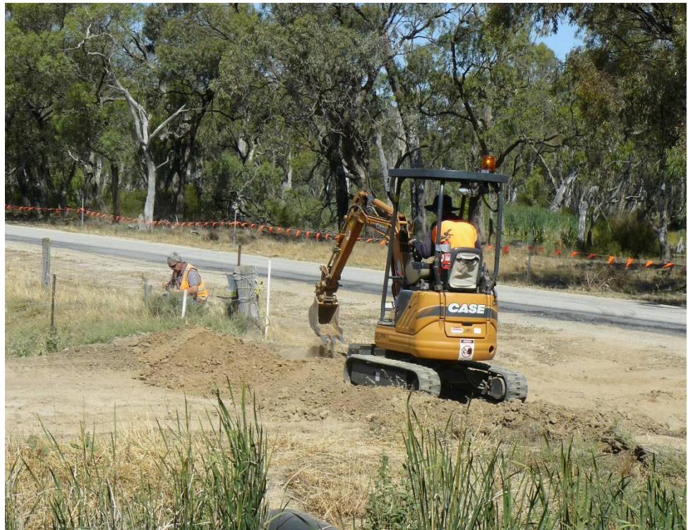
Photo 1: Contractors working to relocate the Telstra cable in December 2012.
