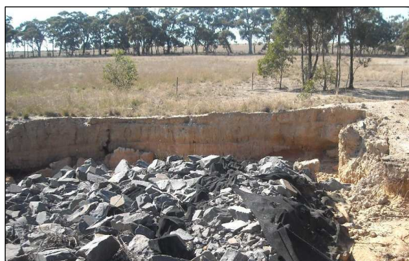
Figure 3: Erosion control structure previously installed by the North Central CMA requiring repair following the extreme flow event. Photo: North Central CMA.
