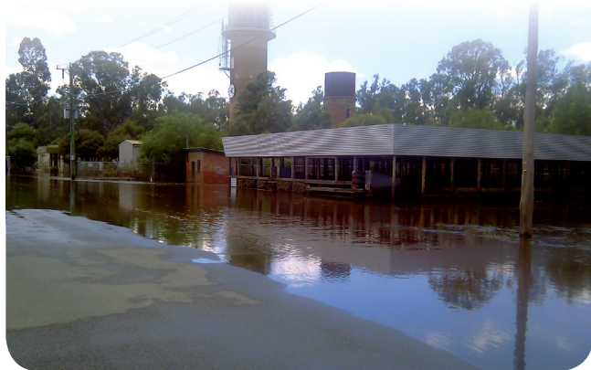
Flood water at Rochester Water Treatment Plant (17 January 2011)
