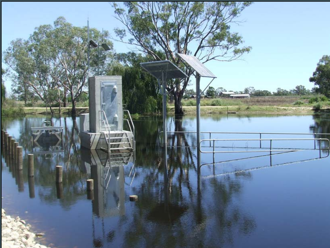
Kerang Fishway during flood, February 2011 (Photo by Tess Grieves)
