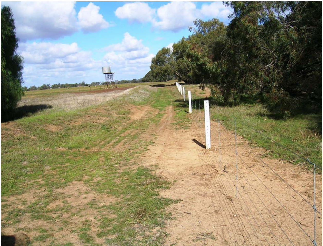
Protective fencing near Boort. Photo: R.Sample
