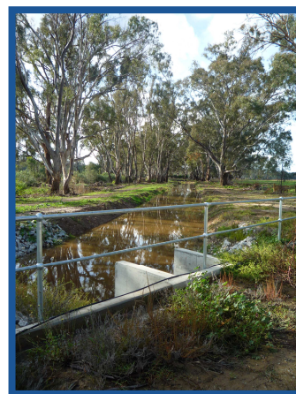
A section of completed primary drain (June 2010)
