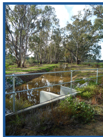
A section of completed primary drain (June 2010)
