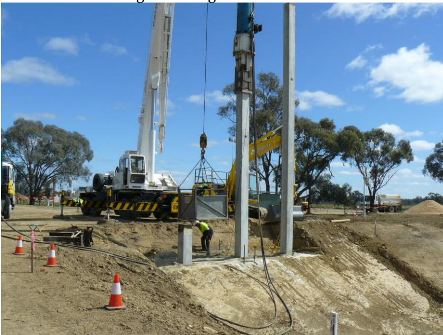
Photo 4: Crane driving piles for new Island Road bridge.
