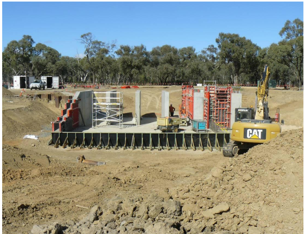
Photo 1: Construction of the Offtake regulator, April 2013.
