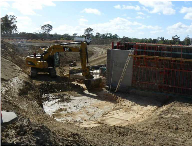
Photo 2: Construction on the Offtake Regulator, April 2013
