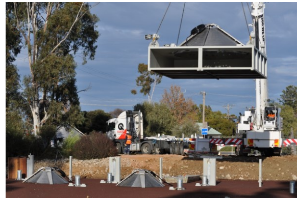
Screen cone being lowered into the creek (Photo: NCCMA)
