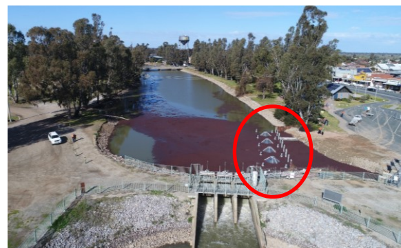
Screen located in front of Cohuna Channel (Photo: NCCMA)
