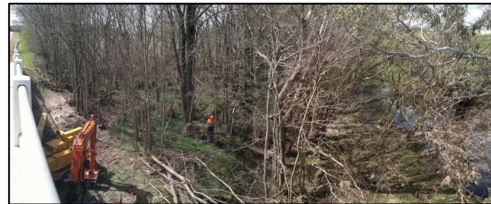
Blockage removal works along Tullaroop Creek, Carisbrook before (above) and after (below). Photo: Platypus Ecological Restorations
