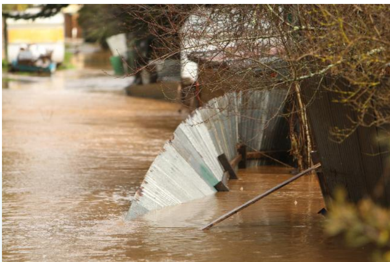
Figure 2- An example of damage to inappropriate floodplain fencing
