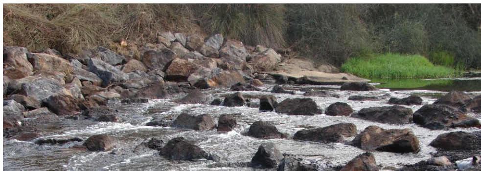
410 TONNES OF ROCK WILL BE USED TO CREATE A FISHWAY AT THE CURRENT WEIR SITE
