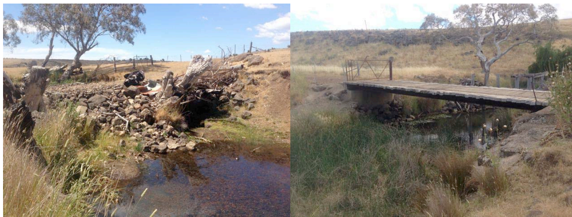
Figure 4. The road crossing at Tourella Estate (left) presents a barrier to dispersal along Birch's Creek whereas the bridge crossing (right) allows free movement of aquatic organisms.
