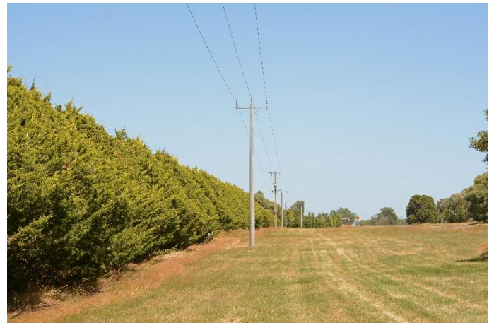
This hedge has been previously pruned by Powercor who recently moved the poles to a new alignment away from the hedge.
