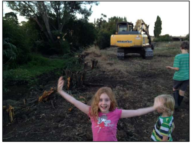
Orlando, Matthaus and Sofia Phillips are excited by the willow clearing works
