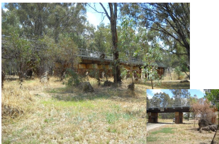
Railway bridge over Campaspe River, north of township
