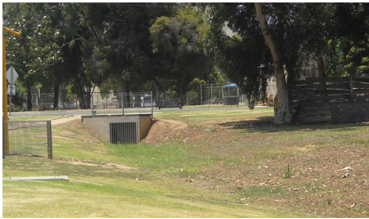
Park – Victoria St/Northern Hwy - Drainage pipe behind bar screen
