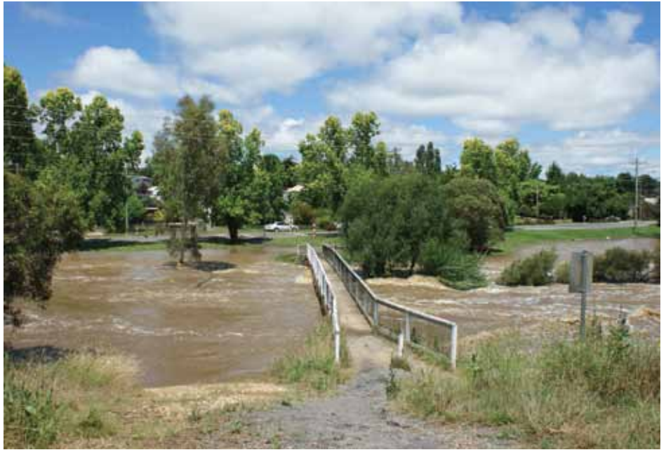
Campbells Creek Winters Ave footbridge in flood, January 2011 Photo: Mal Brown
