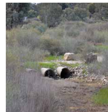
Piped culvert in the Bullock Creek
