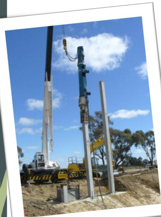
LEFT: Crane being used to construct the new bridge
