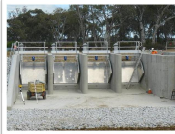
RIGHT: Gates installed on the Hipwell Road Weir
