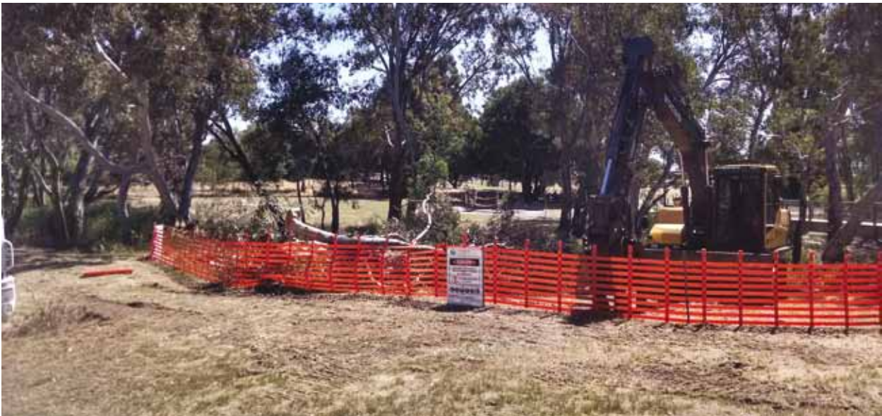
Waterway management works were undertaken at Carisbrook to reduce the impacts of flooding to urban areas. Photograph: Alfred Bouwman, Platypus Environmental Services
