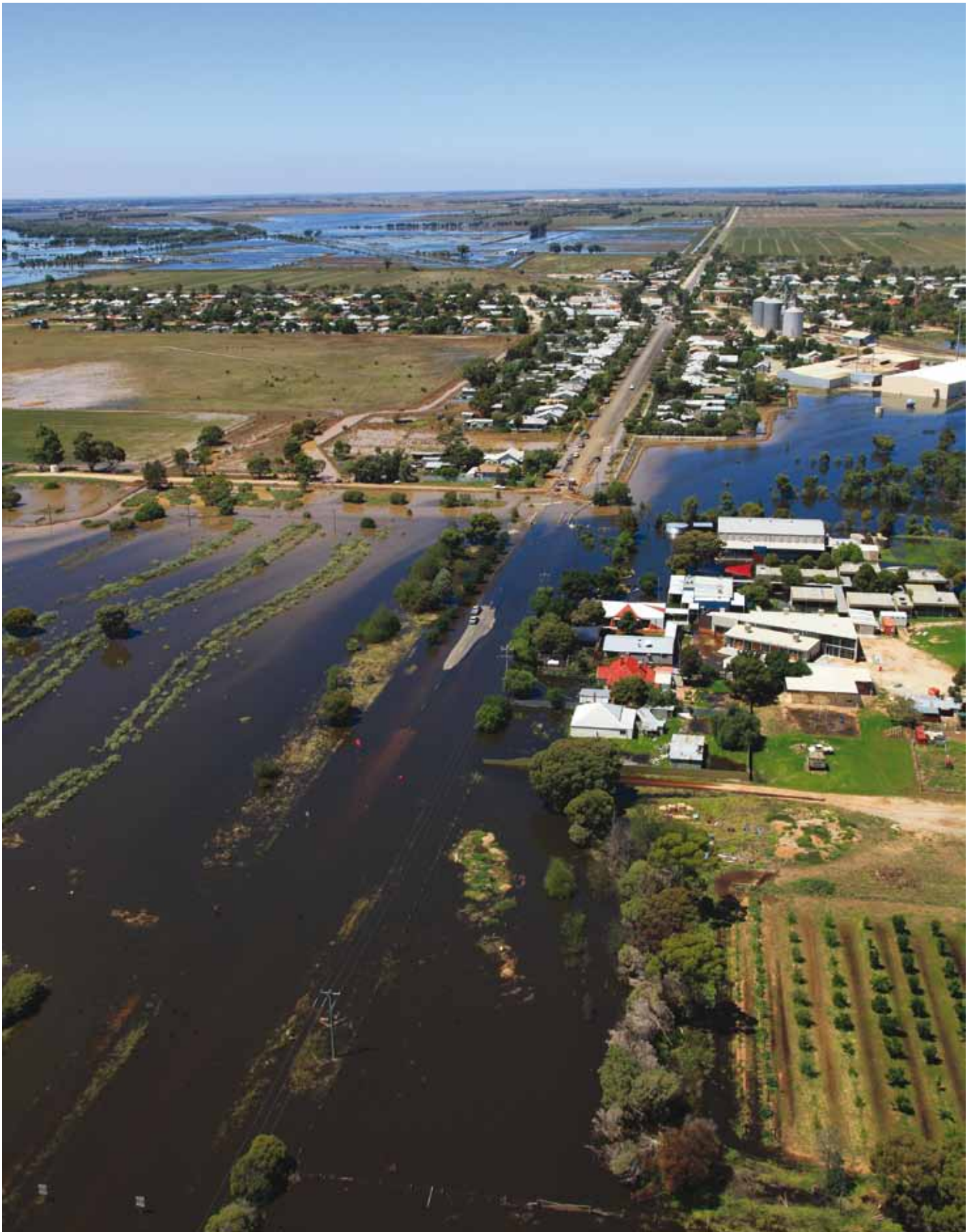
Flooded roads at Pyramid Hill in 2011. Loddon Shire constructed a temporary levee around Pyramid Hill (upper part of the photograph). Photograph: Adrian Martins, North Central CMA
