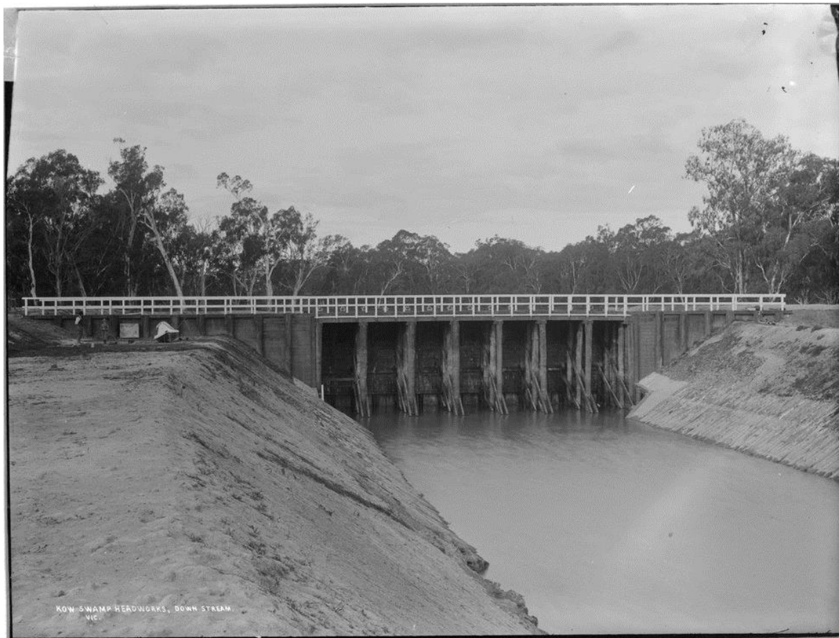
Fig. 6. Original National Channel Inlet Regulator (“Kow Swamp Headworks”) built in 1890. Original photo by State Rivers and Water Supply Commission photographer. Sourced online from State Library of Victoria collection. Out of copyright.
