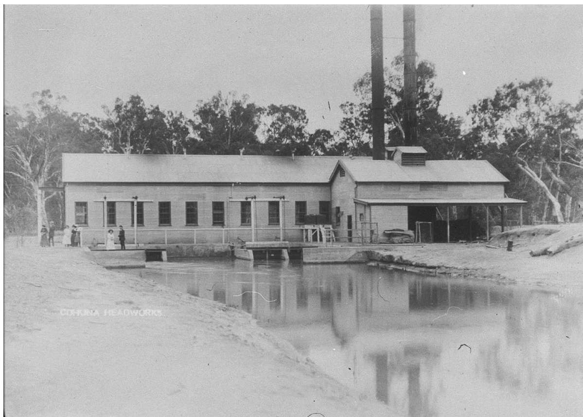
Fig. 5. Cohuna headworks pumphouse in 1914, on the banks of the River Murray close to the Deep Creek inlet. The river is behind the building and the irrigation channel is in the foreground. Photo used with permission: State Library of New South Wales, At Work and Play – 06314.
