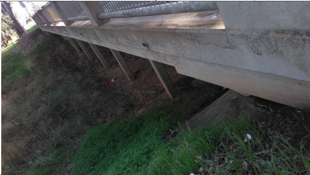
Marong - Serpentine Road Bridge over Bullock Creek. Bridge02
