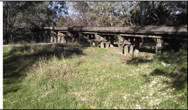
Historic Wooden Rail Bridge
