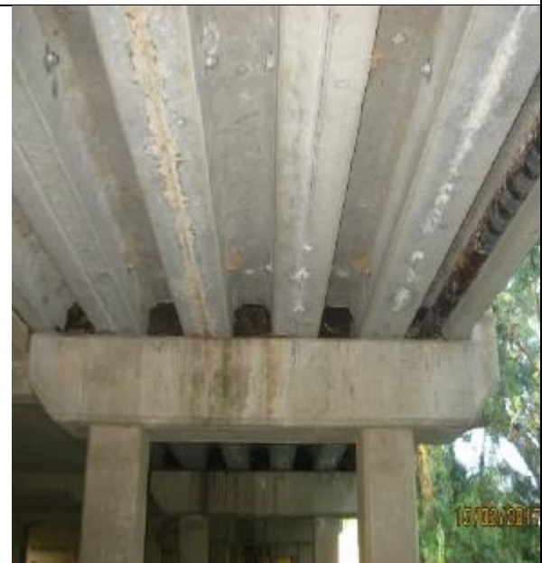
Under – right widening
