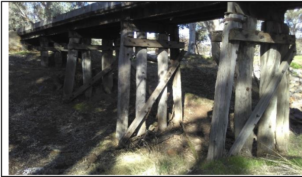
Historic Wooden Rail Bridge
