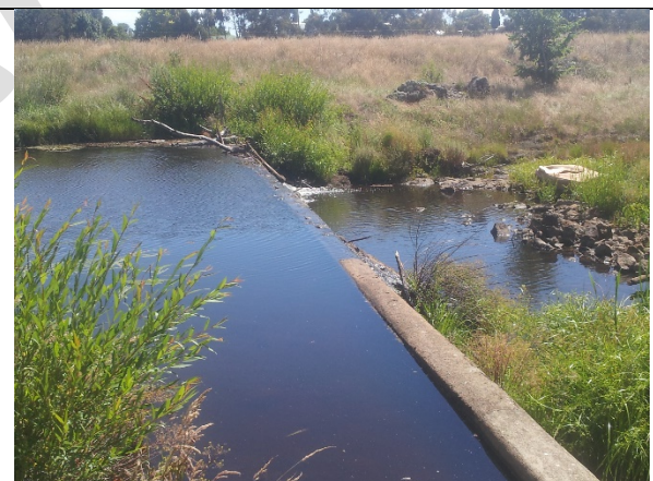
S12 - Hutton Street Weir
