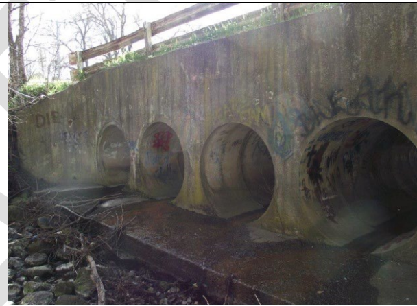
S16 - Ebden Street Culverts
