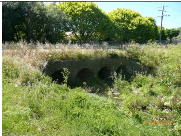
S15 - Mollison Street Culverts
