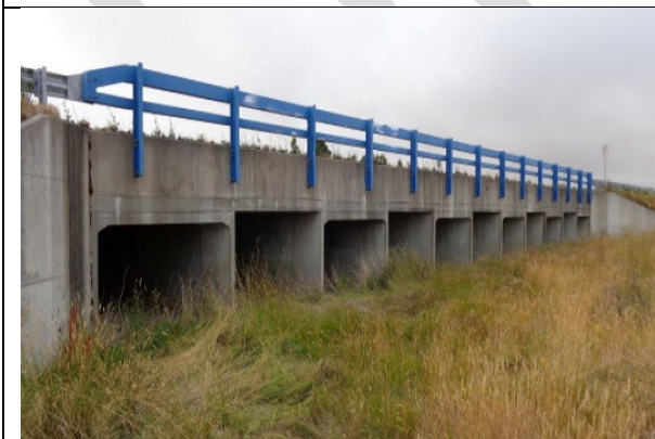
S5 - Calder Highway Culverts
