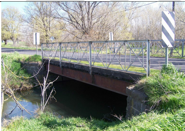
S17 - Wedge Street Bridge
