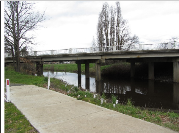
S13 - Piper Street Bridge
