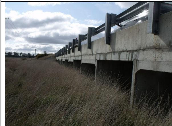
S3 - Carlsruhe Central Road South Culverts
