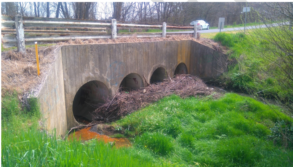
Figure 4-40 Blockage at the Ebden Street culverts
