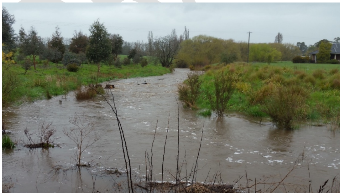
Figure 4-28 September 2016 event looking south-east on Post Office Creek upstream of Wedge Street (refer to Photo 4 in Figure 4-27)
