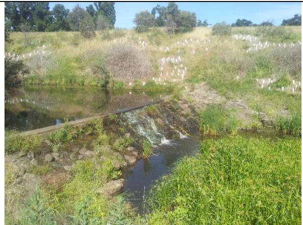
S14 - Campaspe Place Weir
