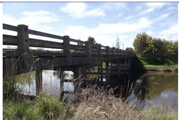
S6 - Cobb and Co Road South Bridge
