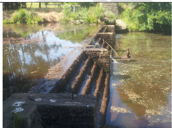
S11 - Greenway Lane Weir
