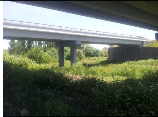
S8 - Calder Highway North Bridges
