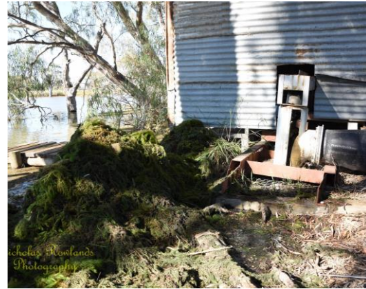
Weed build up around an irrigation pump on Gunbower Creek (Photo: Nicholas Rowlands)
