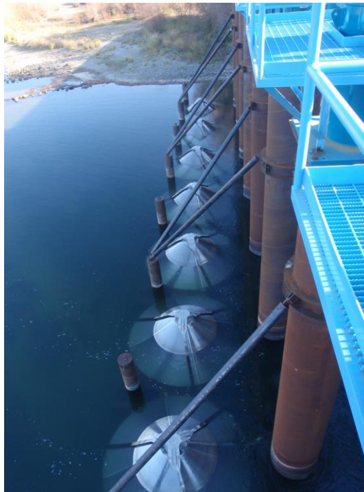
Example of pump screens (Photo: Brett Kelly)
