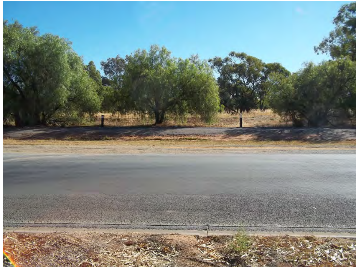
EXISTING CONDITIONS - VIEW 1 LOOKING WEST ALONG BYRNE ST
