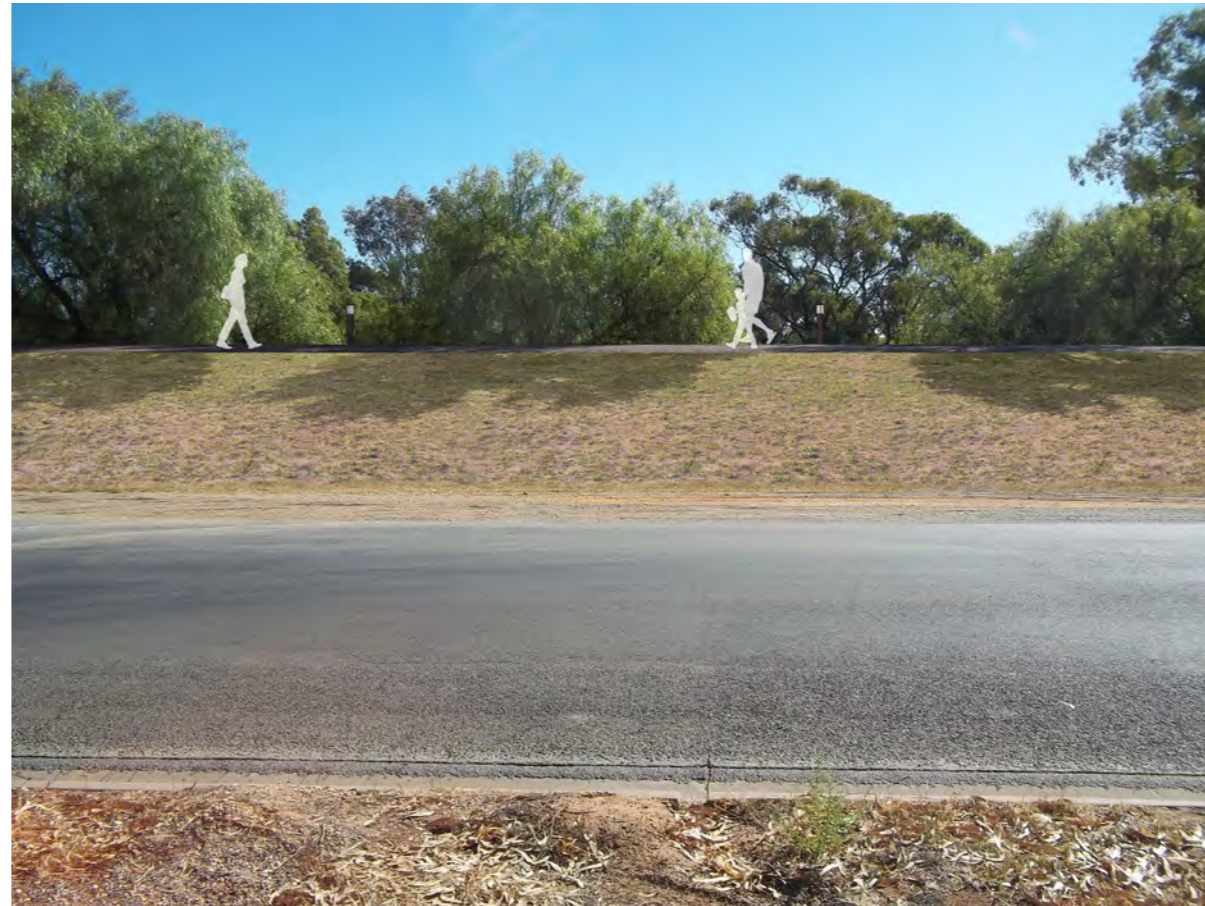
LEVEE 2 - VIEW 1 LOOKING WEST ON BYRNE ST
