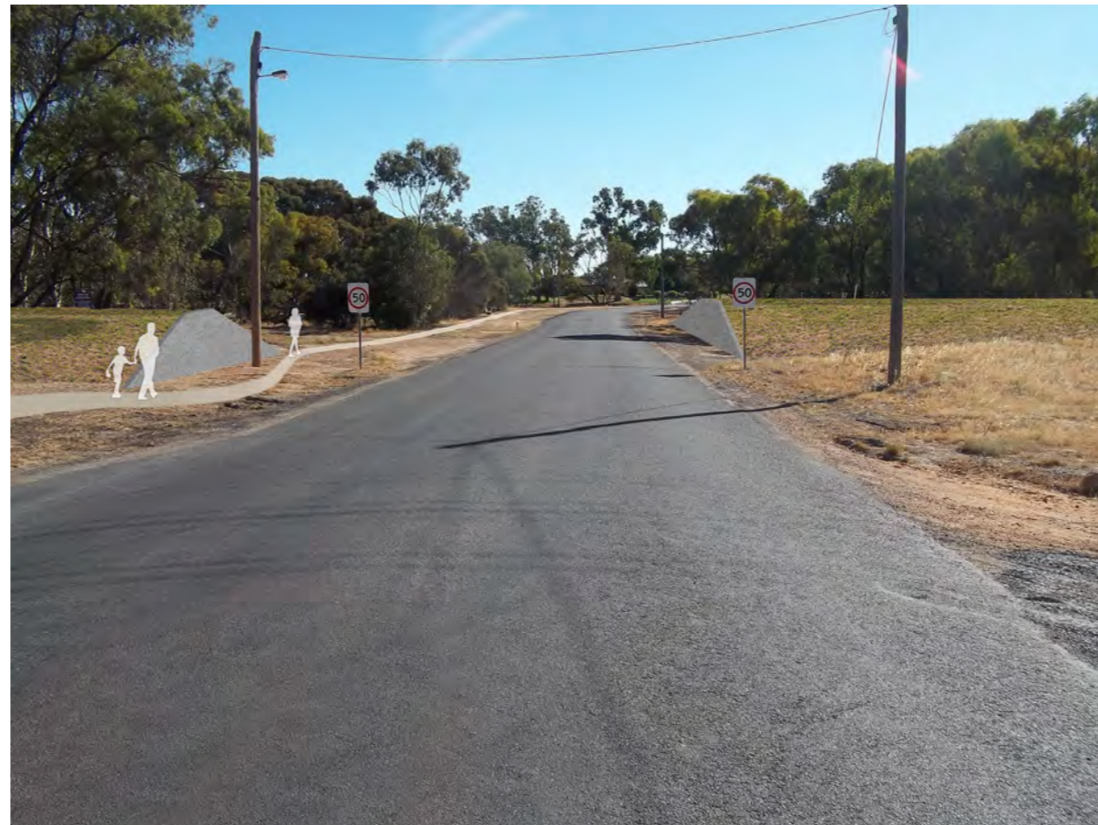
LEVEE 2 - VIEW 2 LOOKING WEST ALONG CAMP ST
