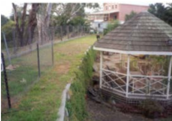
Figure 6-12 Crib Wall Levee
