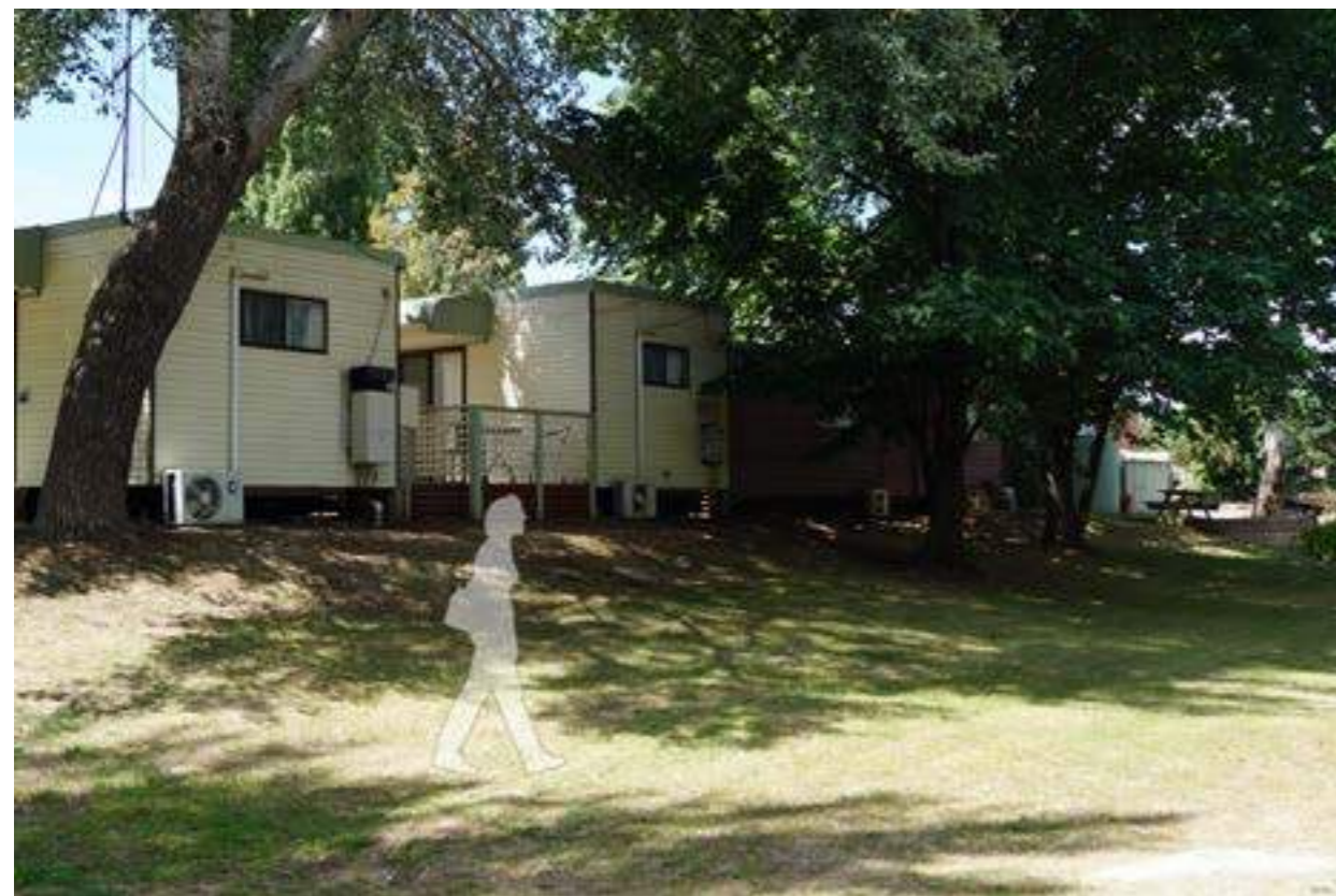
EXISTING CONDITIONS LOOKING EAST AT CARAVAN PARK
