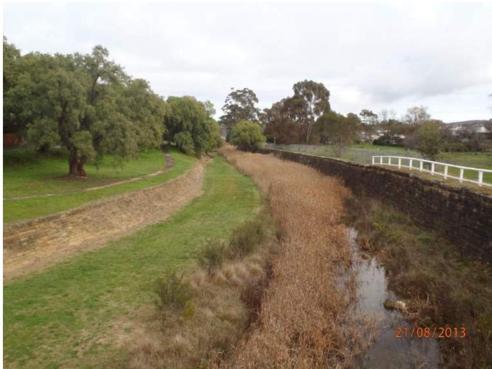
Figure 15 Forest Creek on Leanganook Track Foot Bridge Looking West
