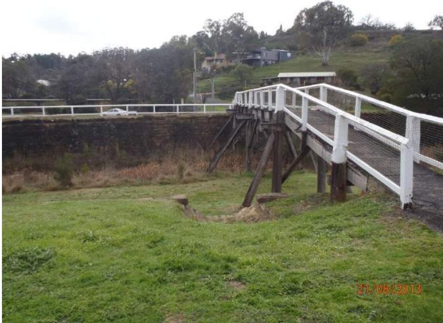
Figure 17 Leanganook Track Foot Bridge
