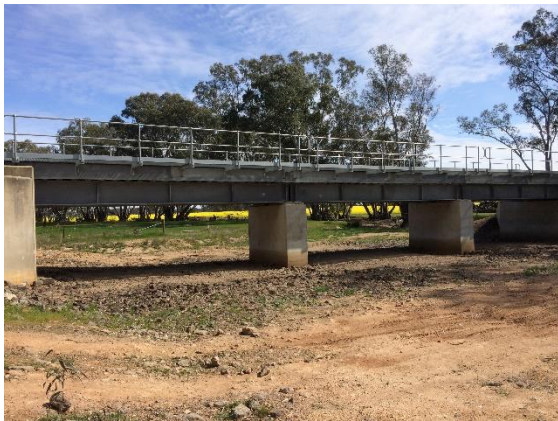
Robinvale Line Rail Crossing over tributary to Bullabul Creek
