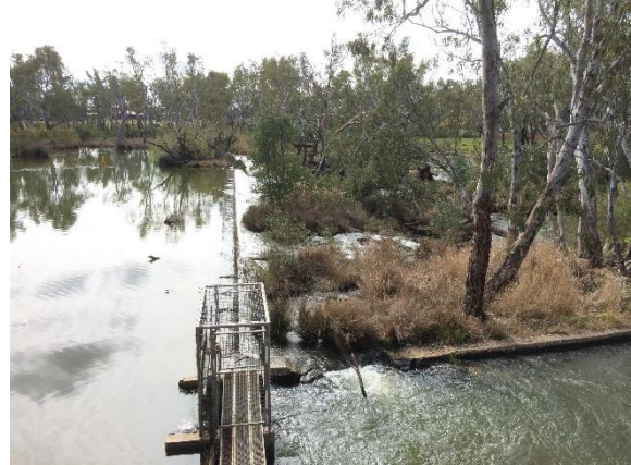
Loddon Weir offtake to Mill
