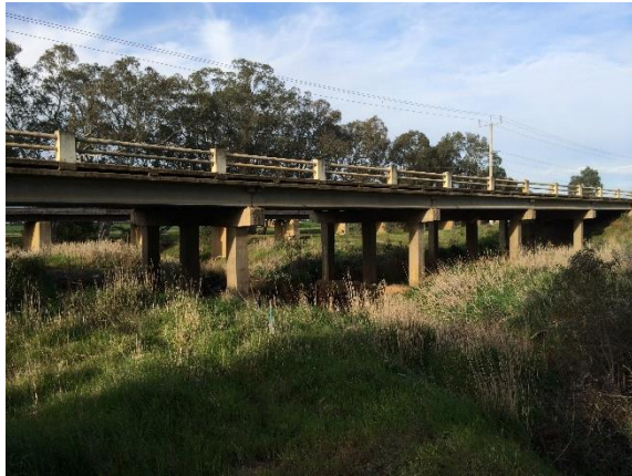
Calder Highway and Eaglehawk-Inglewood railway crossing Bullabul Creek
