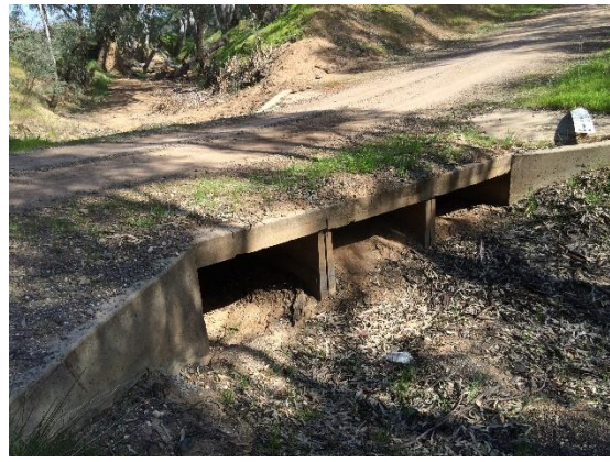
Bullabul Creek Crossing on Black Bridge Road
