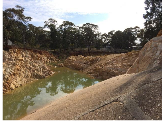
Laanecoorie Reservoir Spillway
