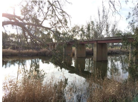
Eaglehawk-Inglewood Line crossing Loddon River
