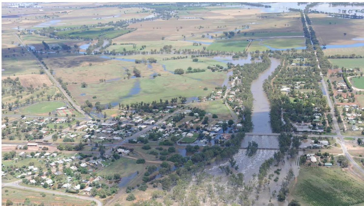
Figure 2-18 Bridgewater flooding 14 January 2011 (Bendigo Advertiser)
