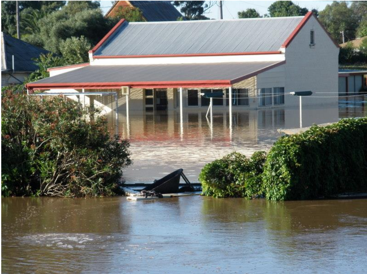
Figure 4-9 Bridgewater Bowling Club close to the peak of the January 2011 flood event
