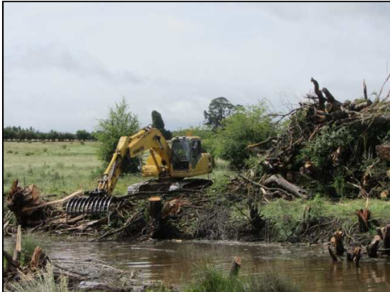
Willow removal in progress (January 2014)
