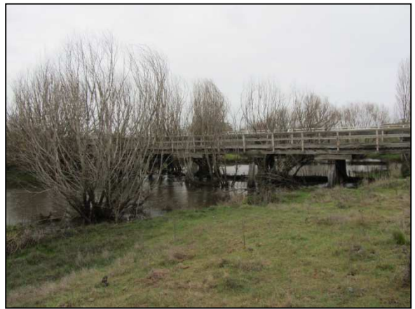
Standing dead willows adjacent to the heritage-listed Windmill Bridge (August 2013)
