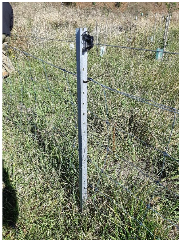
Lay down flood resilient fencing installed across the creek aids stock management while protecting the creek
