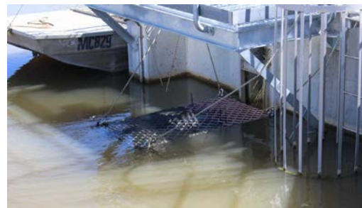
Cage attached to the exit gate of the Hipwell Road fishlock used to monitor fish moving out of the forest
